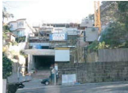
The structure of the block is now complete.
